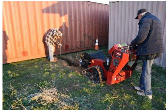
VP Bill guiding the trencher from the brick building to run power. (It saved A Lot of work)
